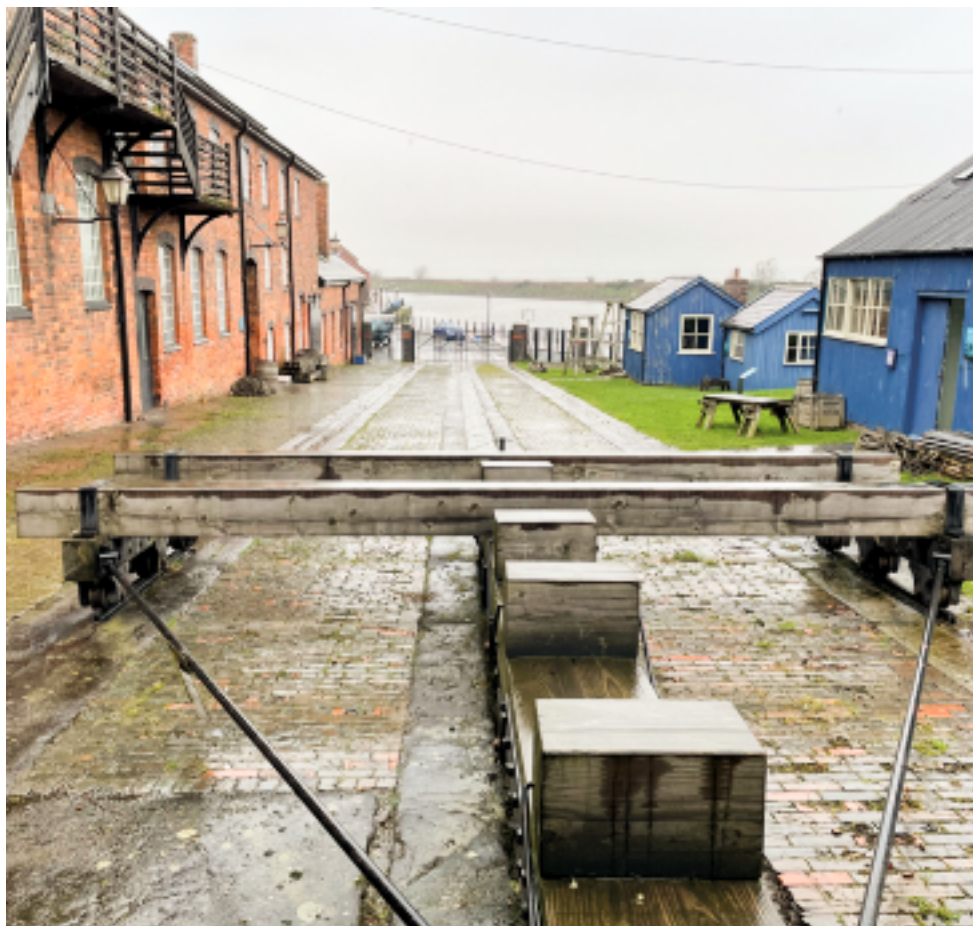
The large slip-way
