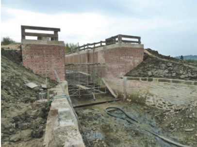
Temporary safety fencing now installed
