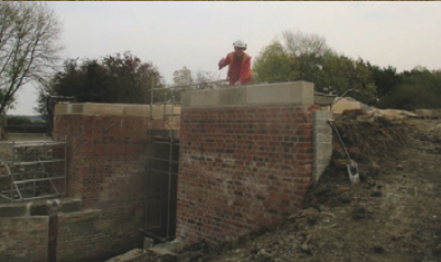
The completed job
