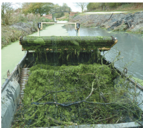
View from Osberton's cab showing the cleared water and in the background the excellent results of the workparties who have opened up the "narrows" between the Bridle bridge and Casthorpe Bridge. Courtesy Ian Wakefield
