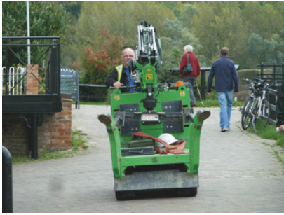
The crane being delivered
