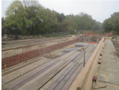
The scaffolding is coming down!
