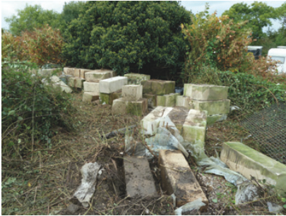
The coping stones - ready for a wash
