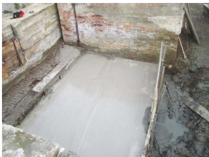
Access cut down to the upstream wing wall to enable a concrete floor (shown left) to be poured for work to proceed on re-pointing and cutting in new stop board recess
