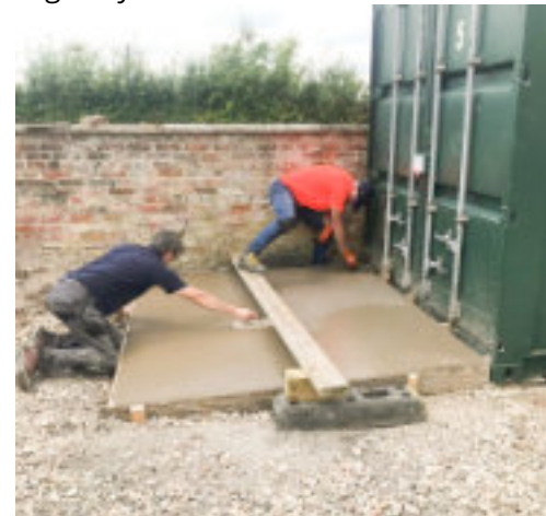
Work on constructing a ramp (22 June 24)
