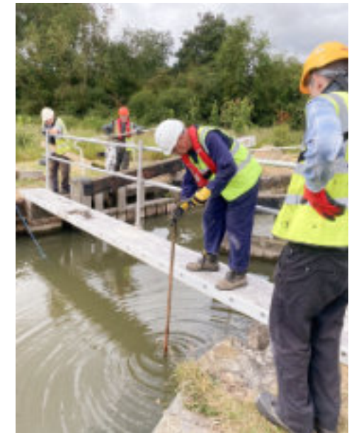
Extract from the Construction Workparty report 28 June 24: Today was a three phase operation: (i) build youngman's bridge (ii) put in stop planks (iii) remove youngman's bridge. All phases completed by the team working in unison. Once the stop planks with tarpaulin were in place John R came to take measurements of the offending paddle.
