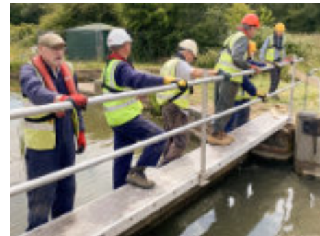
Extract from the Construction Workparty report 28 June 24: Today was a three phase operation: (i) build youngman's bridge (ii) put in stop planks (iii) remove youngman's bridge. All phases completed by the team working in unison. Once the stop planks with tarpaulin were in place John R came to take measurements of the offending paddle.
