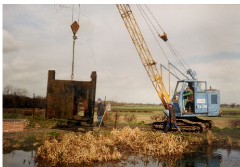
The present top gates, then second hand being installed in 1993.
